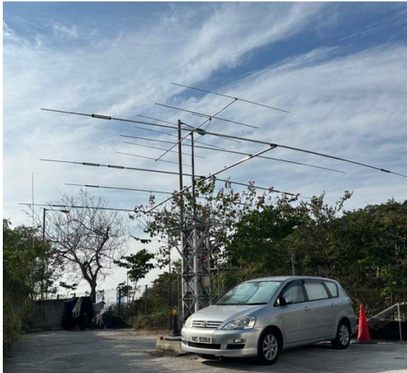
Figure 3 : HF Yagi Antenna
